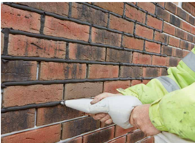
Applying mortar
